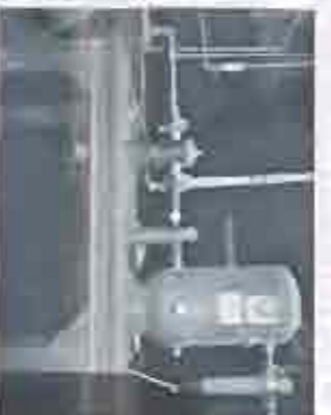
GARDNER-DENVER AIR COMPRESSORS "VAN-AIR" DELIQUESCENT AIR DRYER
